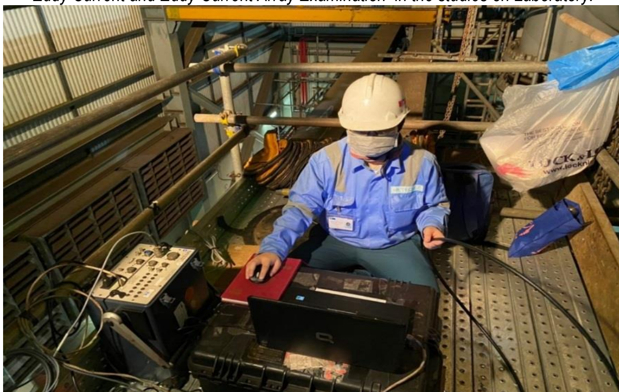
Eddy current Examination for in-service inspection on site.
