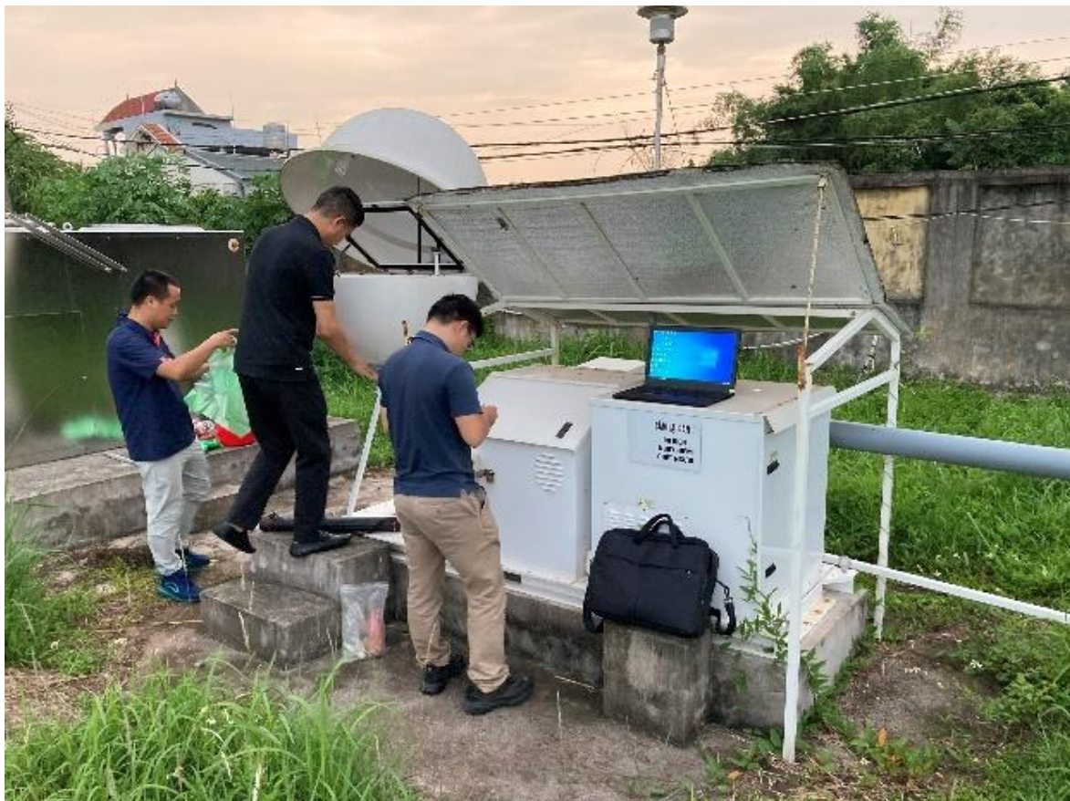
Maintenance of air sampling system at the Mong Cai radiation monitoring station
