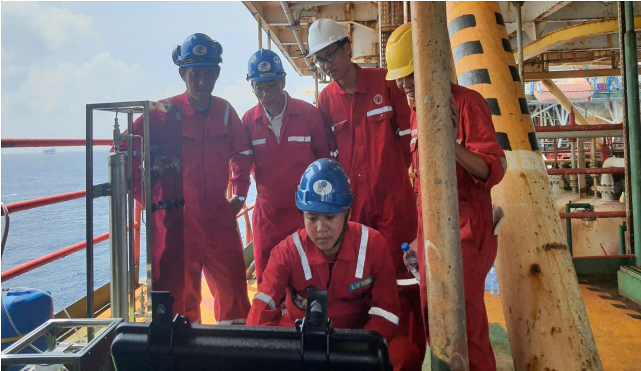
Application of the leak control method for gas-lift wells using the chemical tracer technique
