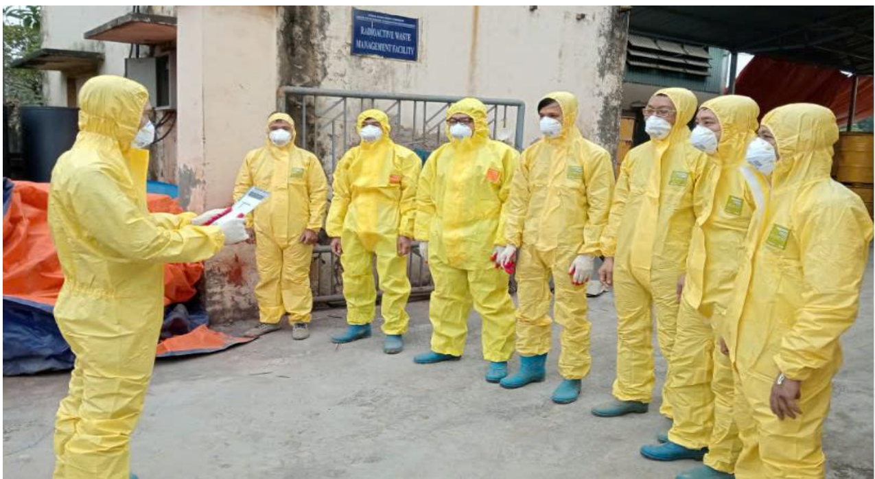
Carrying out the task of repairing the radioactive waste storage facility
