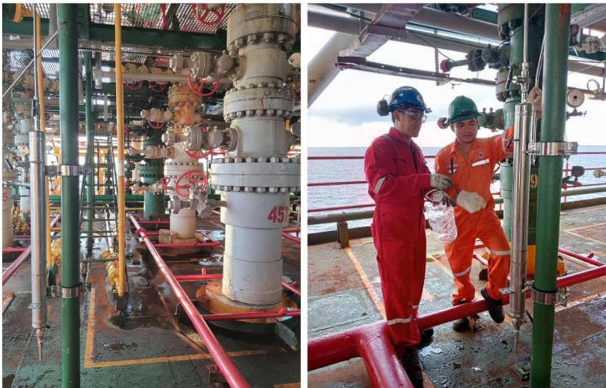
Installation of Well Head Sampler for produced water extraction
